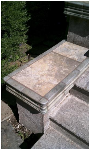
Outdoor stair barrier tile renovation
