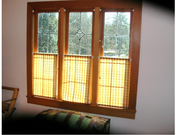
Window completely rebuilt to use existing leaded glass
