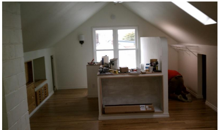
2 nd floor bedroom remodel – bookcase guard rail, reclaimed wood floor, new windows, skylights
