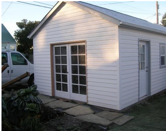
Door jamb made for recycled french doors.
